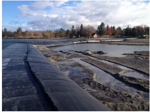
Knutson Dam Project Aqua Dam
