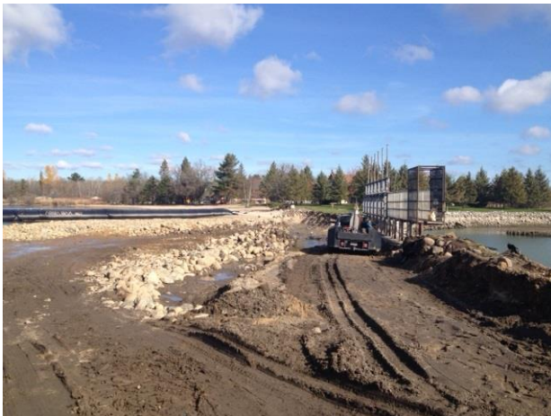
Knutson Dam Project Rock Weir Placement
